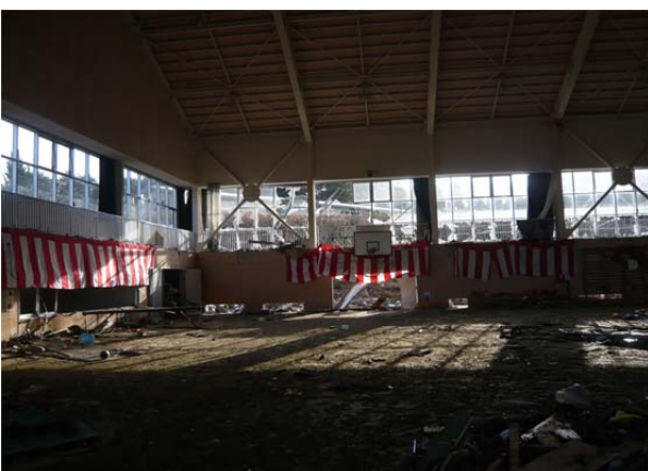
Inside the Gymnasium
